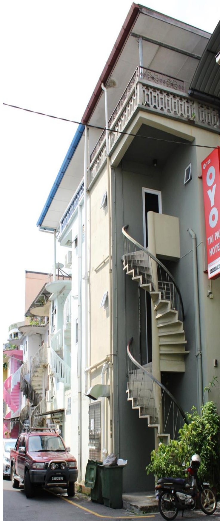
@Padungan Road, Kuching
