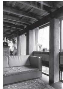
The joists extend beyond the wall line, and are paired with two columns, from which columns hang a continuous row of cabinets as well as a band of windows.
