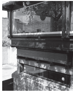
The joists extend beyond the wall line, and are paired with two columns, from which columns hang a continuous row of cabinets as well as a band of windows.
