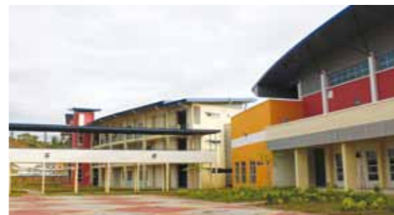
View towards Administrative block.
