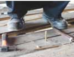
Technique of fixing floor board with a dowel (L-R) : peg the dowel into a pre-drilled hole at an angle; trim the dowel into a ‘V-cut’; drive the cut-off portion into open ‘V-end’ until refusal; trim the expose end with chisel to flush with floor board.
