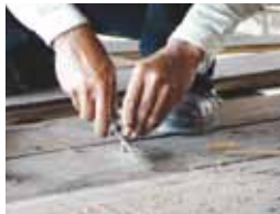
Technique of fixing floor board with a dowel (L-R) : peg the dowel into a pre-drilled hole at an angle; trim the dowel into a ‘V-cut’; drive the cut-off portion into open ‘V-end’ until refusal; trim the expose end with chisel to flush with floor board.
