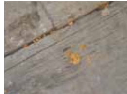
Technique of fixing floor board with a dowel (L-R) : peg the dowel into a pre-drilled hole at an angle; trim the dowel into a ‘V-cut’; drive the cut-off portion into open ‘V-end’ until refusal; trim the expose end with chisel to flush with floor board.
