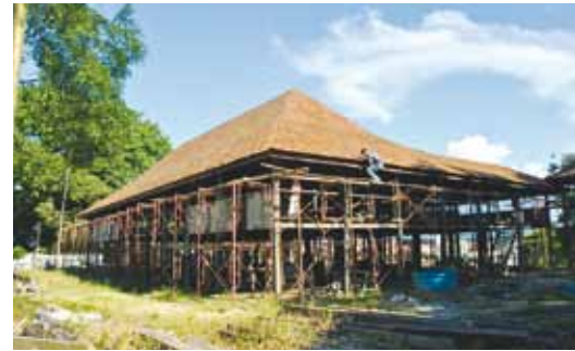
Roof and wall cladding works in progress in May 2014.
