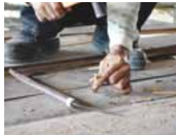
Technique of fixing floor board with a dowel (L-R) : peg the dowel into a pre-drilled hole at an angle; trim the dowel into a ‘V-cut’; drive the cut-off portion into open ‘V-end’ until refusal; trim the expose end with chisel to flush with floor board.
