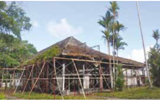
Stabilizing the dilapidated building before dismantling in June 2013.
