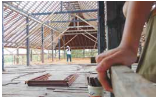
Re-construction of structure and roof frame in March 2014.
