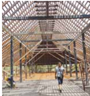
(L-R) First floor interior, before and after laying of ‘belian’ shingles.
