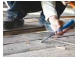
Technique of fixing floor board with a dowel (L-R) : peg the dowel into a pre-drilled hole at an angle; trim the dowel into a ‘V-cut’; drive the cut-off portion into open ‘V-end’ until refusal; trim the expose end with chisel to flush with floor board.
