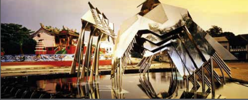
Kuching Waterfront's Hornbill Fountain - Designed by Conybear Morrison, this fountain represents, "Birds in Flight". Constructed of riveted stainless steel sheets supported by structural stainless steel pipes, which also carry water.
