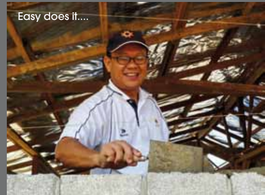
3 barrows of sand + one bag of cement + 8 buckets of water.
