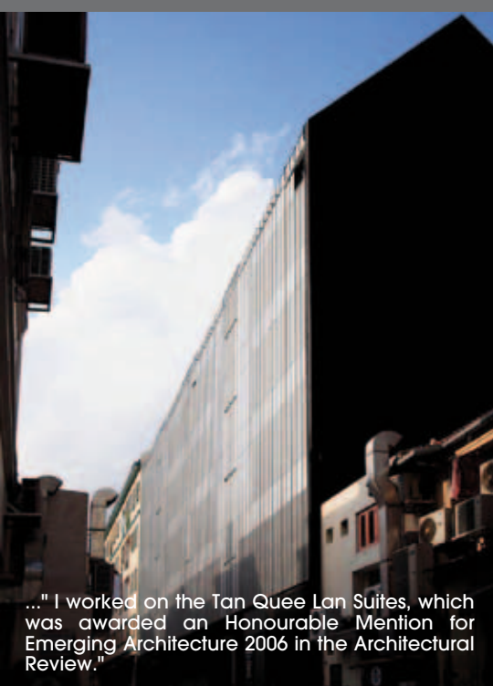
"The architectural concept allows for a contrast between the old conservation shopfront façade and the rear new lightweight steel structure separated by a series of courtyards."
