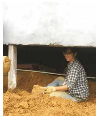
Digging the holes for new pad footings at the building's rear.
