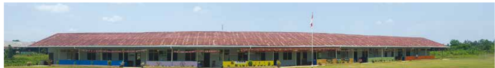
The existing primary school building.
