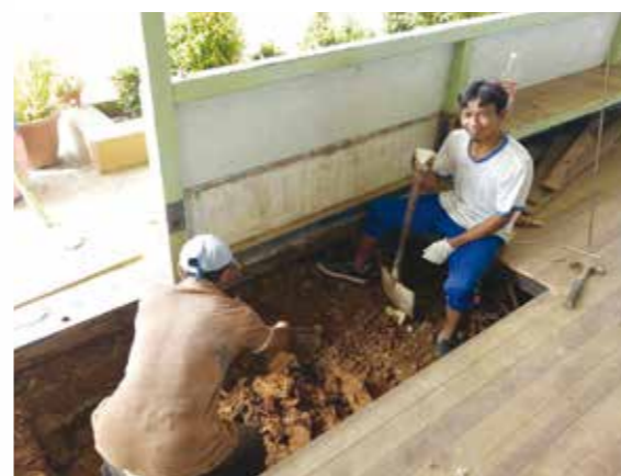
Digging the holes for new pad footings at the building's rear.
