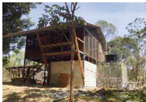
Rebuilding - flood resistant housing module in Dabong Kelantan.
