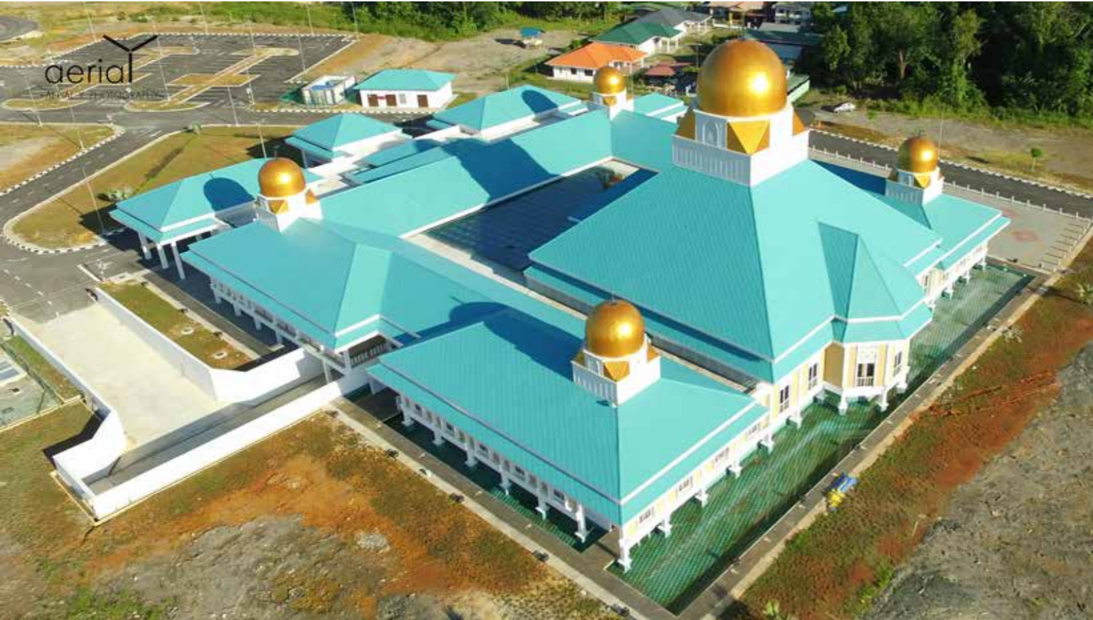
Aerial view of Masjid Darul Hana, Kuching
