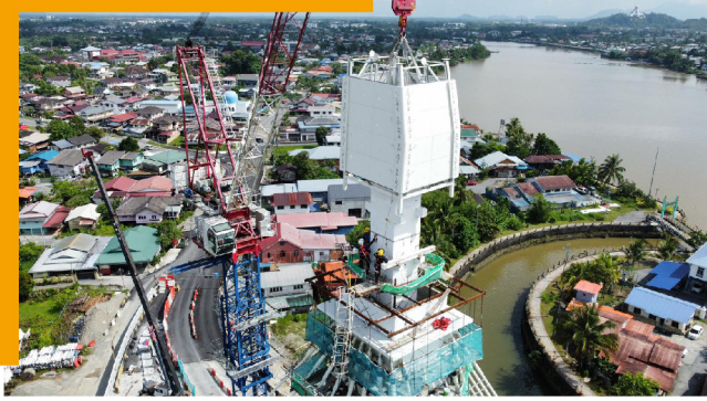
Cladding installation on the top part of the mast
