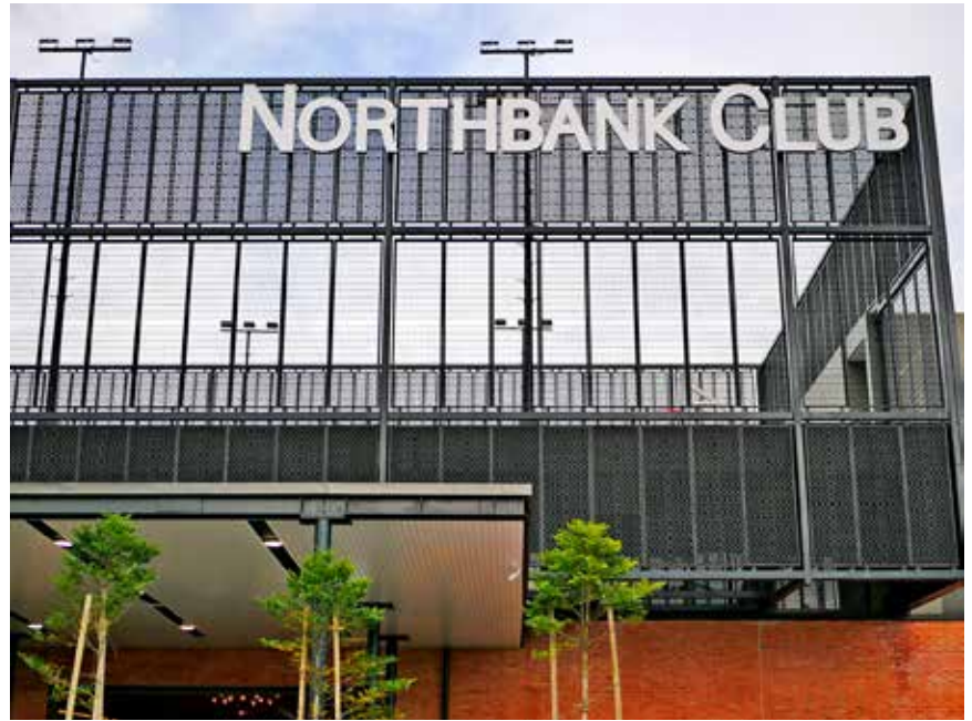
Screens constructed of steel frames with irrigation mat and versatile fencing infills form the enclosure of the rooftop outdoor multi-court; they also shield the facilities on Level 2 from the western sun.
