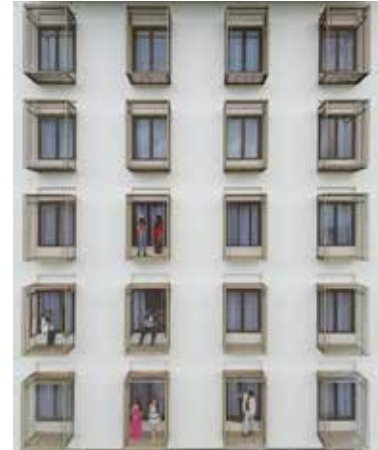
The 'pods' were added to give the guest rooms an outdoor component, as well as farcade treatment.
