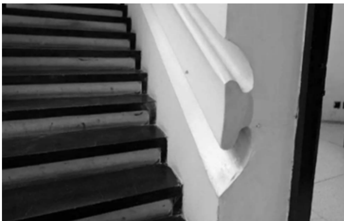
Stair to mezzanine.
