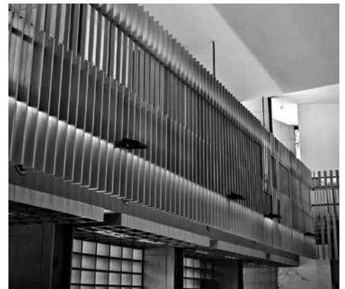
Occasionally, site visit at the end of construction: Recalling "I told you so it's nice moments", appraisal and satisfaction (in earnest hope).
