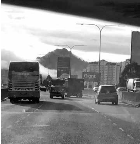
6.30am - On my way to a farm house project around Sang Lee, we are going to start demolish an existing timber house.
