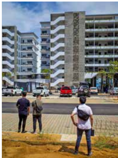
Vent blocks and off form walls as facade design material palette.
