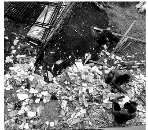
3.00pm - We clean up the debris and move them to the garage.
