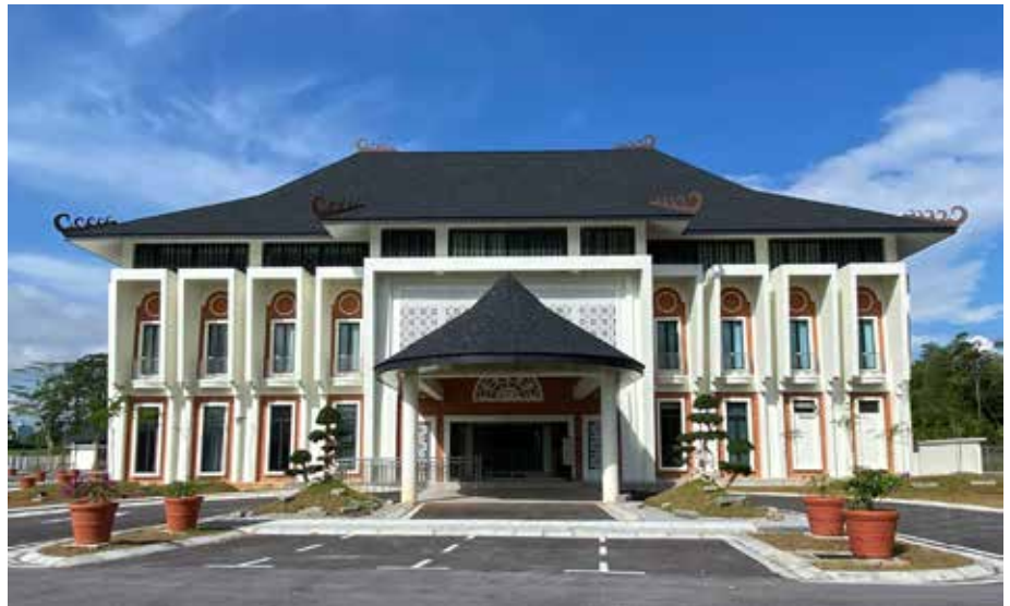
Admin Block Front Entrance.
