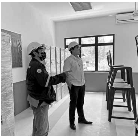
2:00pm - inspecting the mock-up of a classroom recently completed by the contractor.
