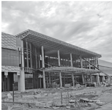
1.00pm - Inspection on the composite panel installation at a factory at Samajaya Industrial Park.
