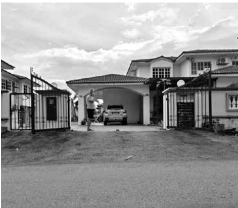
Site visit before construction: sometimes visual surveillance is more effective than measured ones, but involves climbing and bending.
