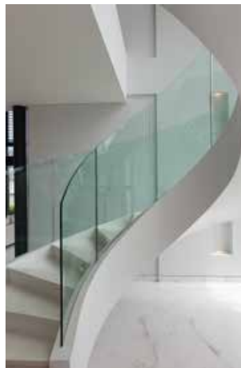
Spiral stair expertly crafted from steel plate, an homage to the family's years of expertise in ship building.
