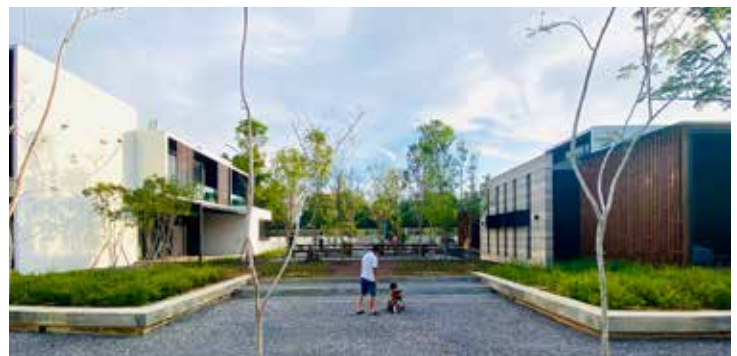
A central courtyard hones the balance and tension between the pair of houses; both accepting, both unrelenting.
