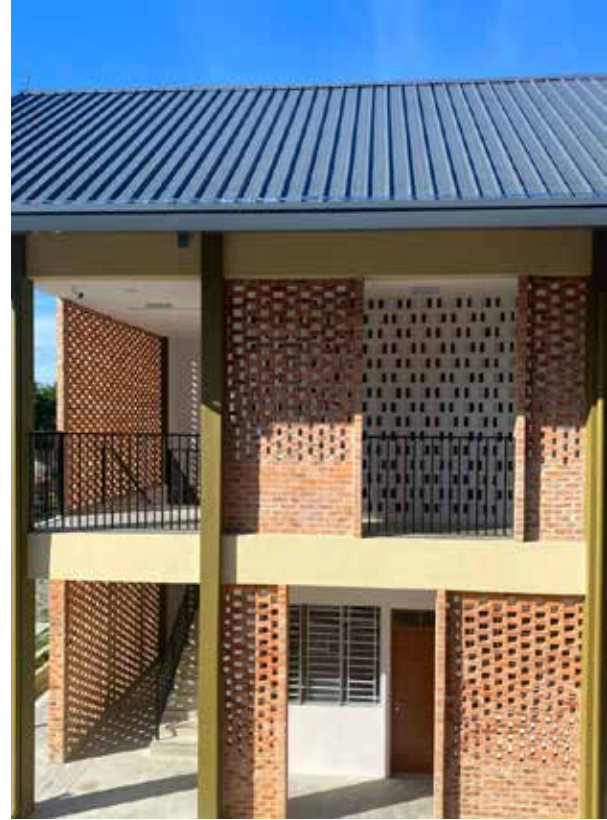
Exposed brick screening.
