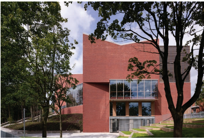
O'Donnell & Tuomey's Lyric Theatre in Belfast (2011) was built to a tight budget, with its function expressed in the form and materials selected and crafted to weather well with age. ( Photo Credit : DENNIS GILBERT )
