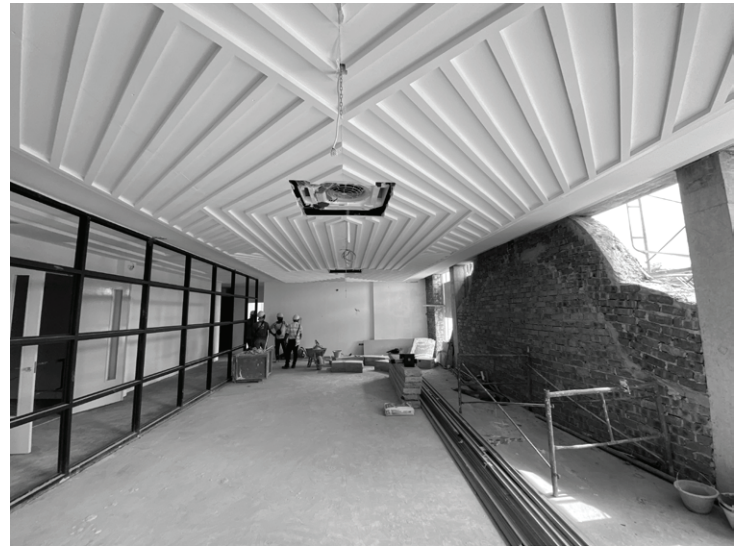
Admin Meeting Room under construction.
