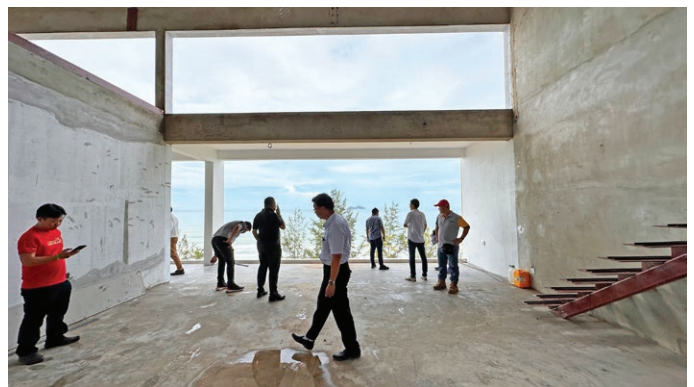
Site inspection at penthouse unit.
