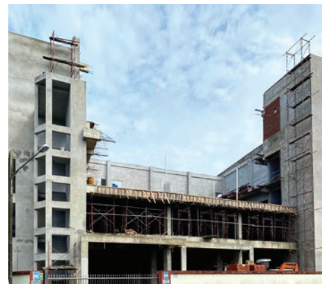
The stage 2 of structural works can only commence after the mobile crane removed from the middle of the building.
