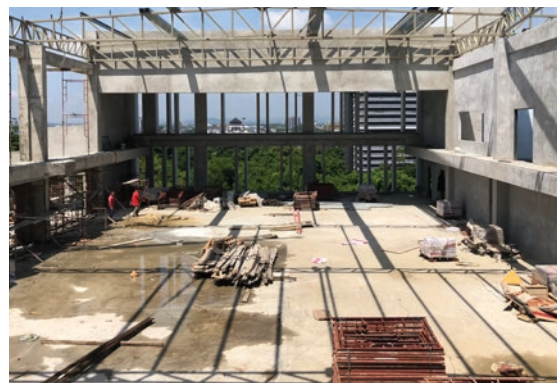
Top floor before main roof covering.
