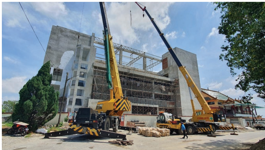
Installation of roof trusses in progress.
