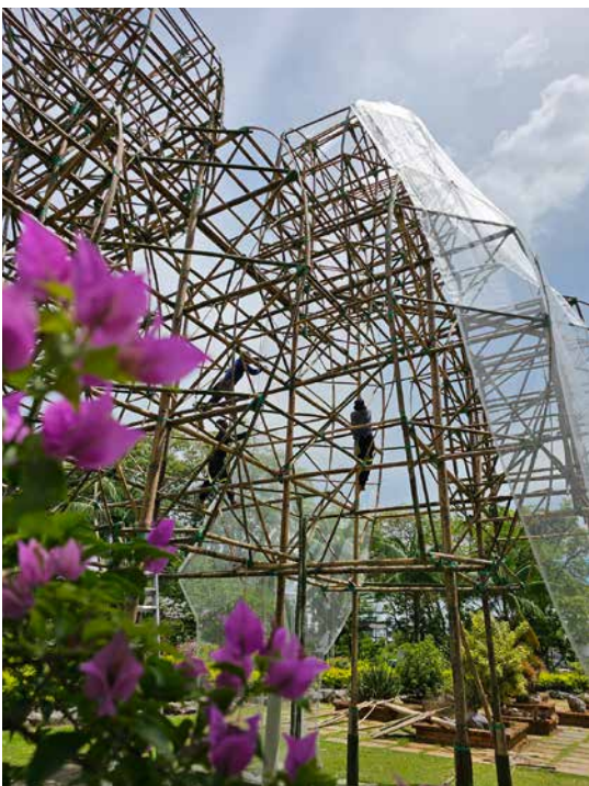
Structure veiled an woven with agriculture netting, creating a soft aesthetic.
