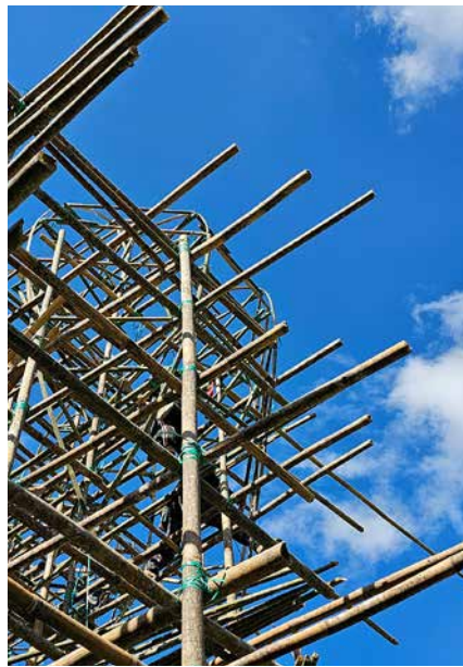
Assembling the bamboo framework: from simple grid to intricate design.
