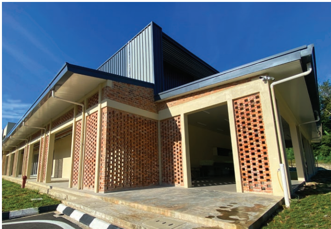
Multipurpose Hall Verandah Screening.
