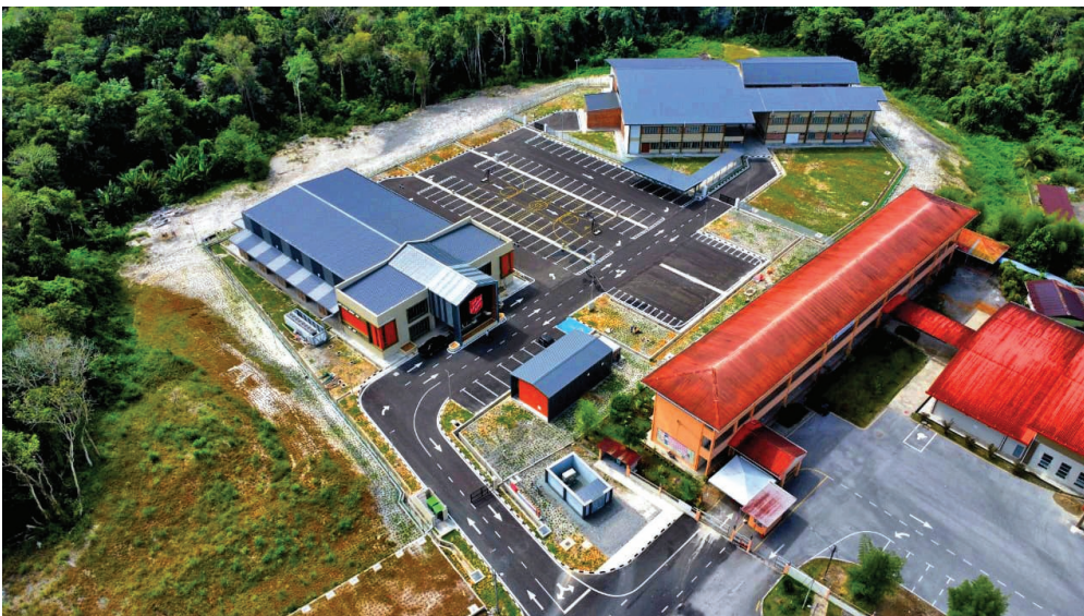
Aerial view of The Salvation Army Home with SJK Chung Hua Sungai Jernang next door.
