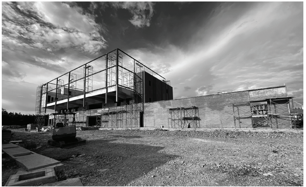
Construction of the enclosure of the rooftop outdoor multi-court.
