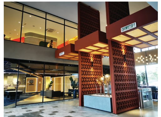
Main entrance and lobby.
