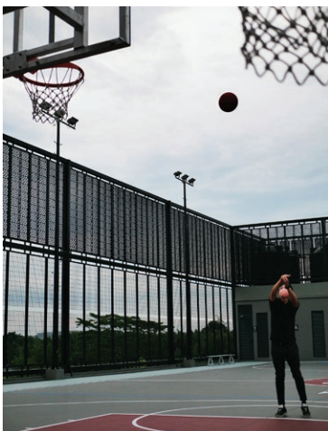
The rooftop Outdoor Multicourt acts as the 'fifth' elevation.
