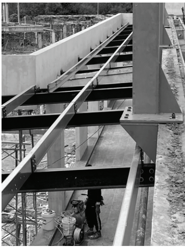
Steel frames for the outdoor multi-court.
