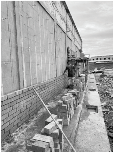
Construction in progress.
