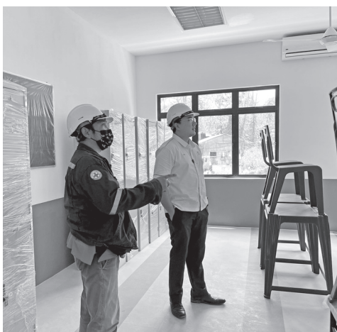
2:00pm - inspecting the mock-up of a classroom recently completed by the contractor.
