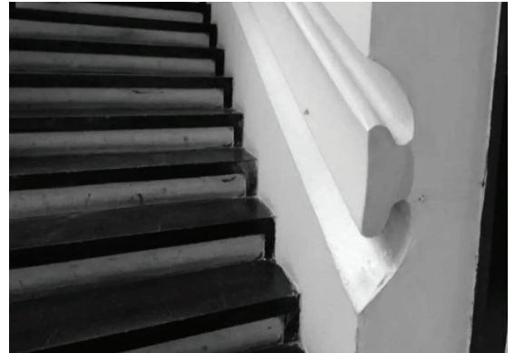
Stair to mezzaine.
