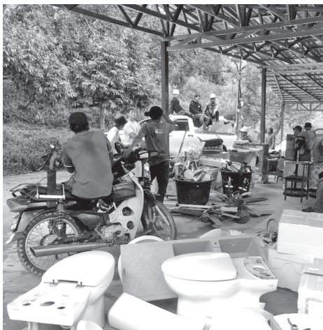
5.00pm - 6.00pm - Sending all the debris out for proper disposal.
