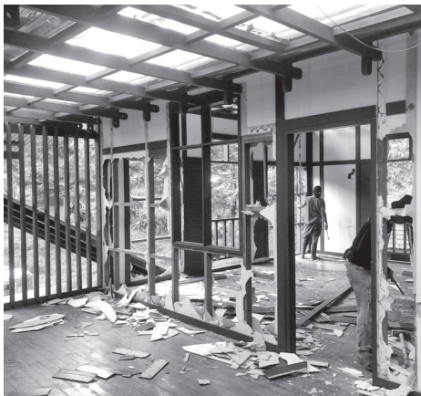
9.00am - The farm workers have started dismantling electrical appliances, GI conduits, window & door panels, toilet fittings to reuse and we sort out the timber based on sizes.
