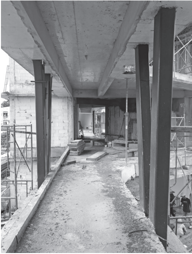
Decorative Steel Column at Connecting Corridor.
