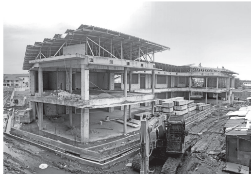
PRA School under construction.
