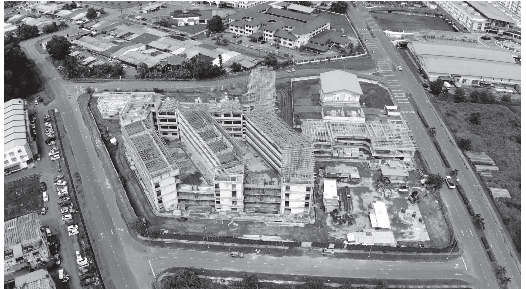
Left aerial view of construction site.
