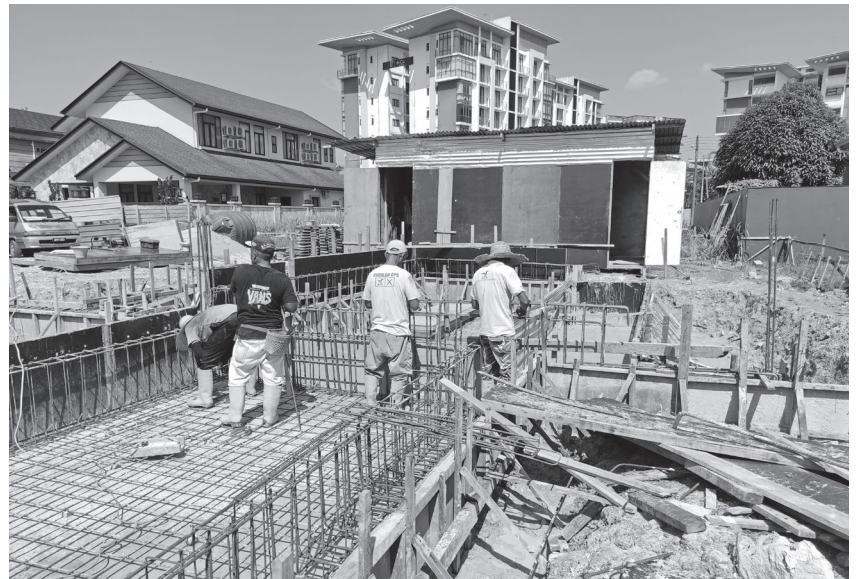
Sub-structure works in progress.
