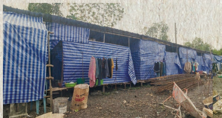
Blue canvas building - Chat equates the makeshift structures of the construction sites and temporary structures of migrants to the vernacular architecture of the past, because they suited life in the tropics and local culture. The blue plastic walls can be 'peeled back' to create a window for the inhabitants who would do most of their activities on the floor.
