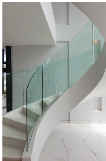
Spiral stair expertly crafted from steel plate, an homage to the family's years of expertise in ship building.
