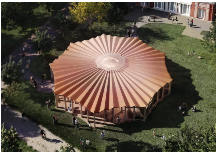
The Serpentine Pavilion 2023 design is shaped to avoid the surrounding tree canopies and roots, becoming structured like a leaf. (Lina Ghotmeh Architecture, Courtesy Serpentine)
