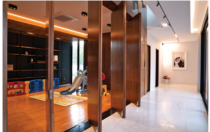
A homogenous circulation is made possible by the installation of the timber pivot doors.
