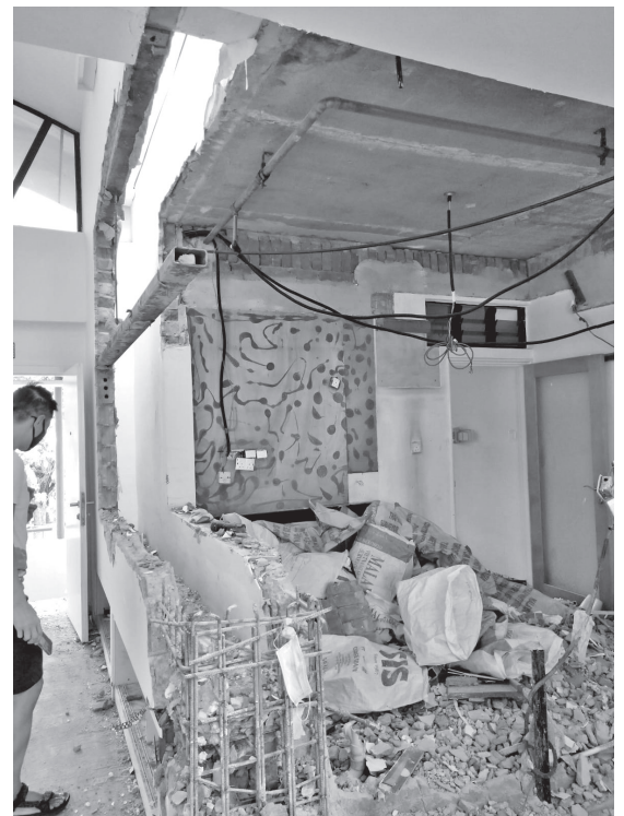
Construction in progress
