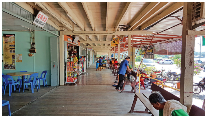
The Old Bazaar corridor.
