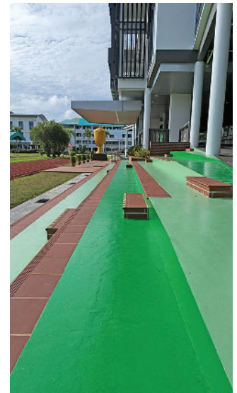
Building with amphitheatre step seating design alongside the existing 100m running track.
