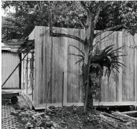
2.30 p.m. TV room extension - inspecting recently struck concrete wall.
