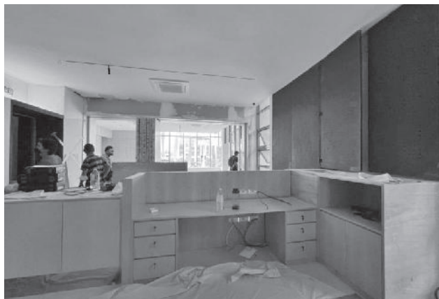
Furniture & lighting installation. (13.06.2022)
