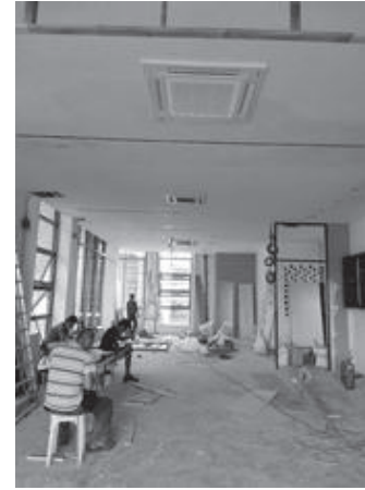
M&E WORKS - Installation of air-cond & wiring cabling above ceiling completed.
