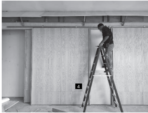
SEMINAR ROOM - Installation of plywood sliding panel with perforations motif.
