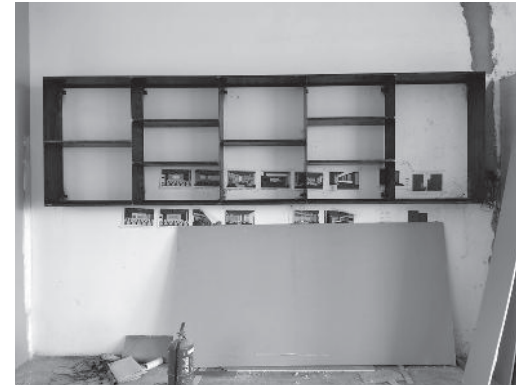
RECEPTION & LOUNGE - Mild steel shelving installed next to entrance.
