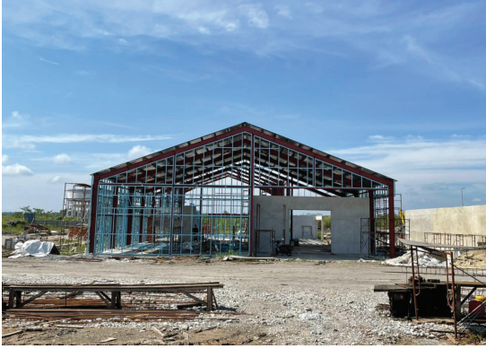
Portal frame steel structure taking shape.
