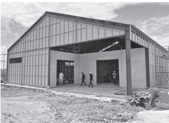
External wall for most area is made of corrugated metal cladding externally and insulated cement board internally.
