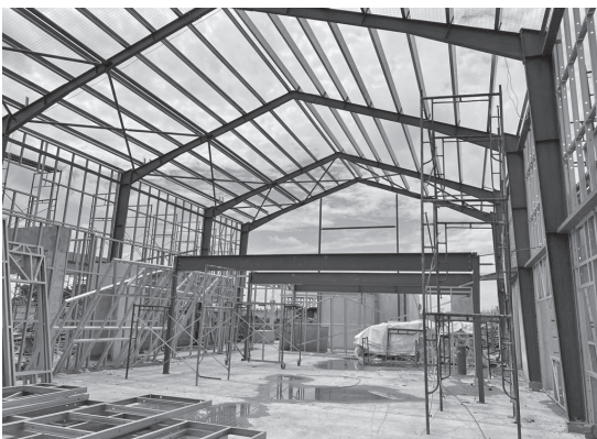
Interior view of the portal frame steel structure.
