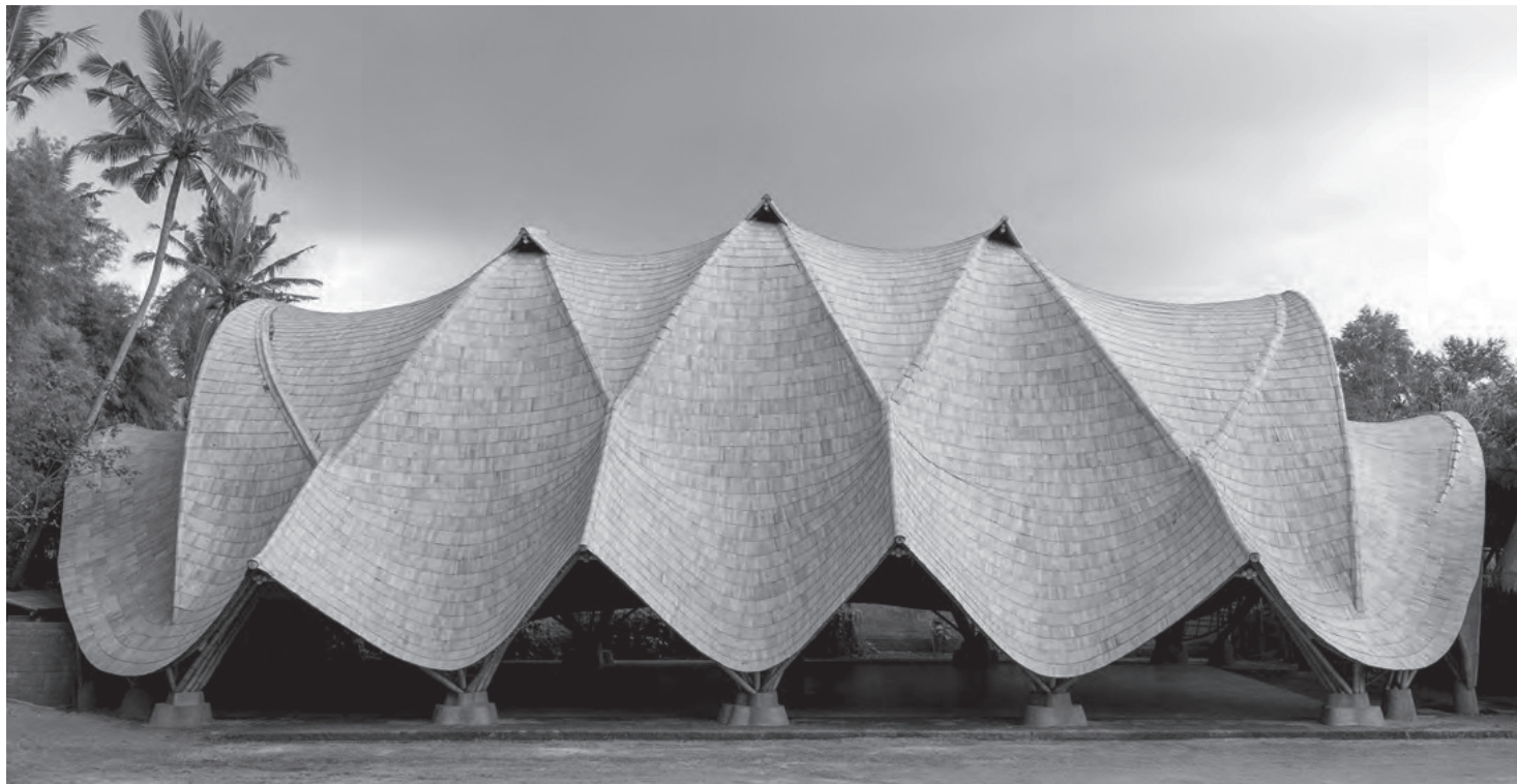
The Arc Building at the Green School, Bali, Indonesia is designed in bamboo with arches spanning up to 19m. Designed by IBUKU in collaboration with Jorg Stamm and Atelier One. (Photo by Tommaso Riva)
