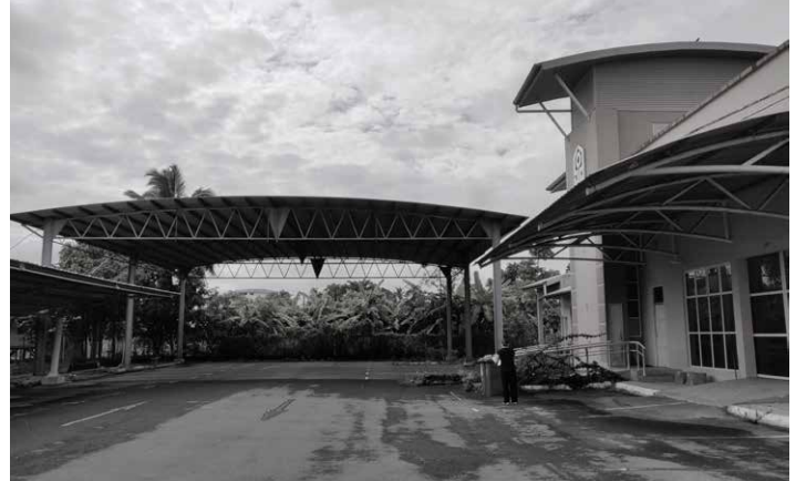
The original building when view from the street - it was the offices and showroom for a car dealership.
