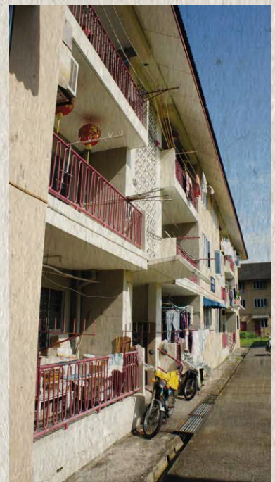
The simple act of turning up the floor beam serves as a balustrade at the same time.
