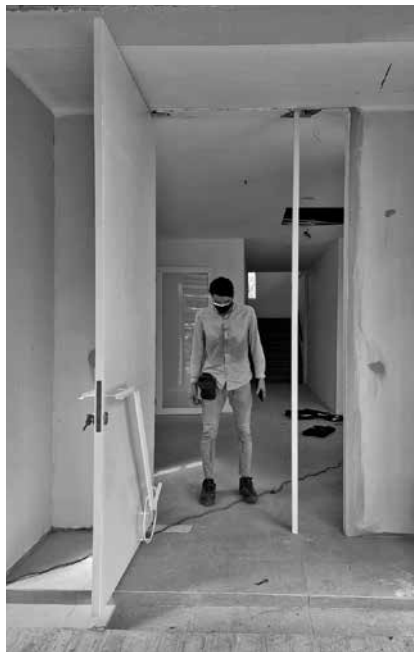
Under construction - Ah Teck testing out the floor hinge.
