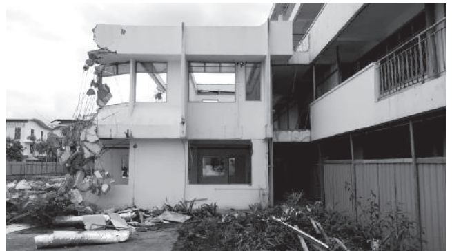
Demolition work begins.
