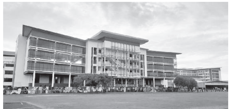
Installation of Aluminium works.
