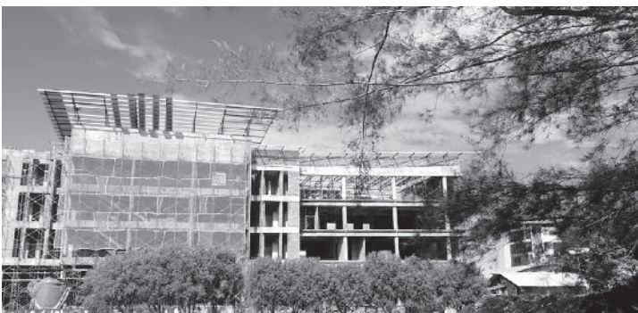
Construction of Roof Canopy.
