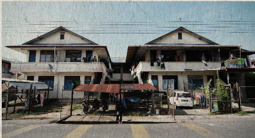
Front elevation from Jalan Bukit Assek.
