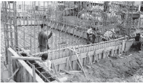
Construction of Lower Ground Floor (below existing ground level).
