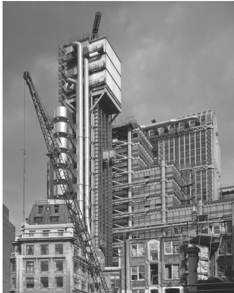
1980s: Lloyd's Building, City of London; Richard Rogers Partnership. (Credit: Martin Charles, RIBA Collections)
