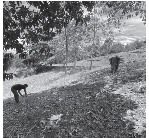
2:30 p.m. Overseeing setting out for a CSR project at Greccio retreat centre.
