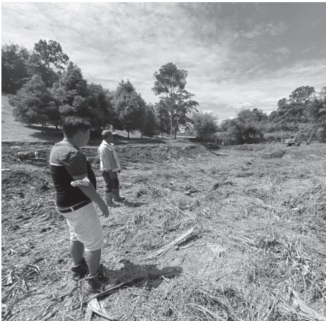
10:00 a.m. 'Hakka' translator for client to site clearing contractors.
