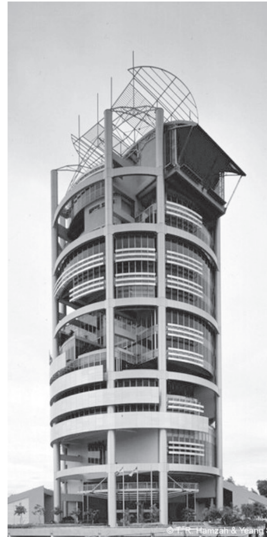
Menara Mesiniaga bioclimatic tower, designed by TR Hamzah & Yeang and completed in 1991 near Kuala Lumpur.
