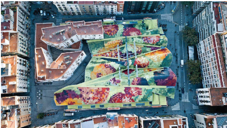
Santa Caterina Market, Barcelona, designed by Enric Miralles Benedetta Tagliabue Architects. Credit: MBT. CHEN ZHANG / ALAMY STOCK PHOTO
