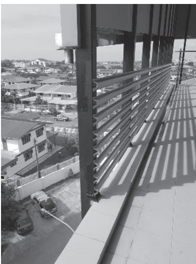
Construction of Top Span Handrail.
