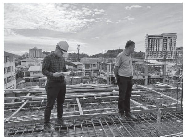
Inspection by Engineer and Employer.
