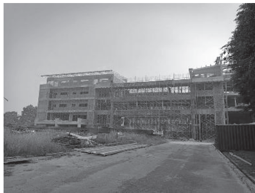
Construction of Roof Mezzanine.
