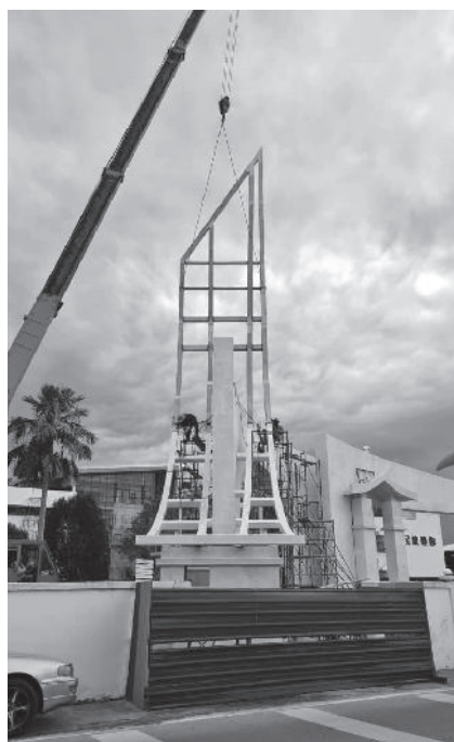
Construction of School Gate Roof.
