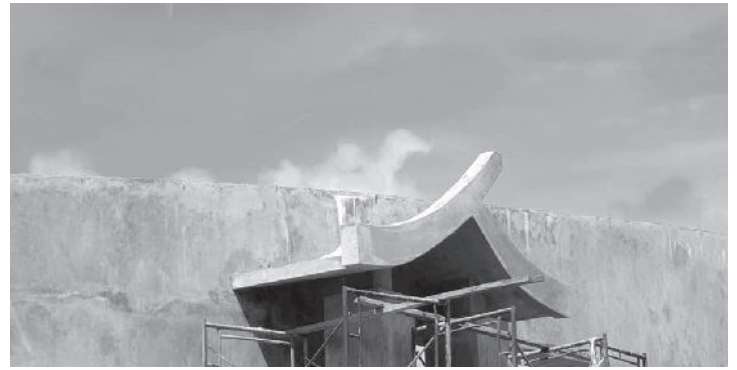
Construction of Roof Fin.
