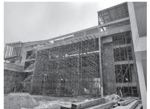
Construction of Front Facade.
