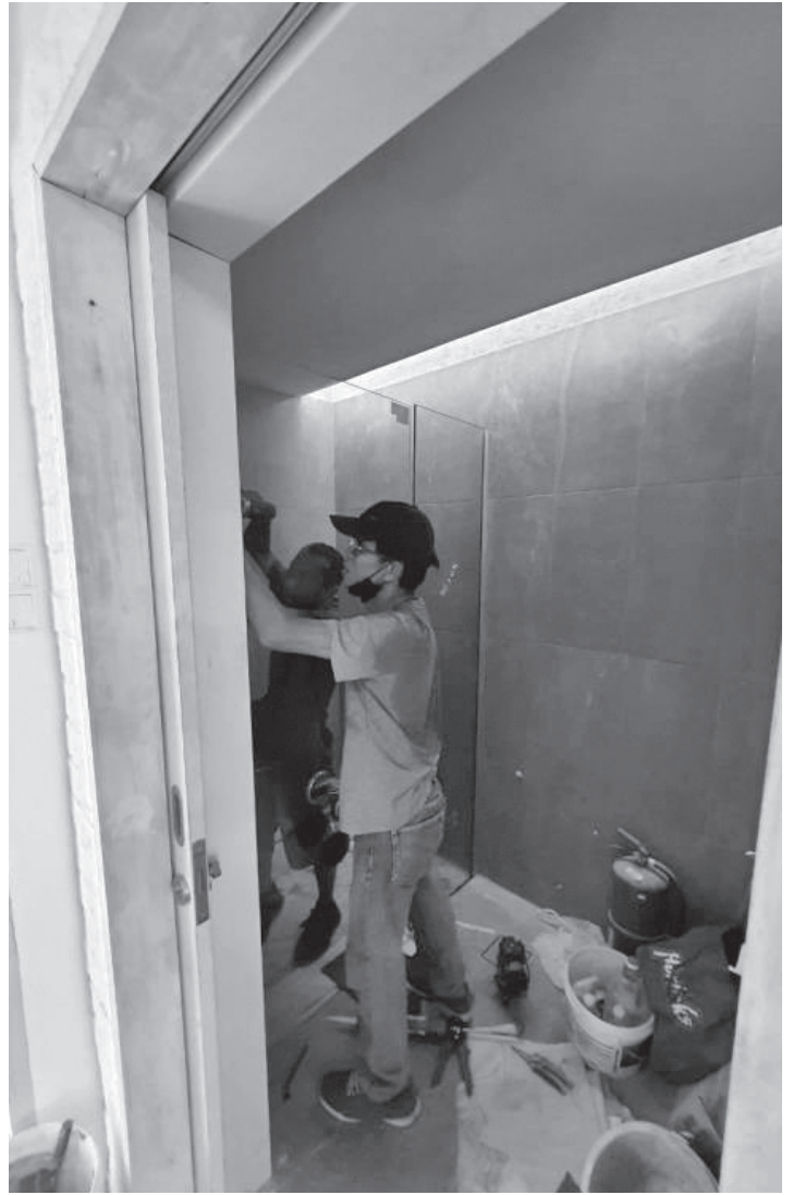
Shower glass installation. (12.06.2022)
