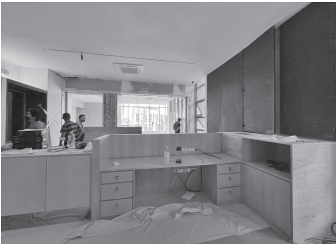
Furniture & lighting installation. (13.06.2022)
