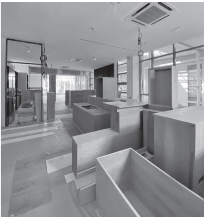
Built-in furniture being mobilized to site. (09.06.2022 - 10.06.2022)
