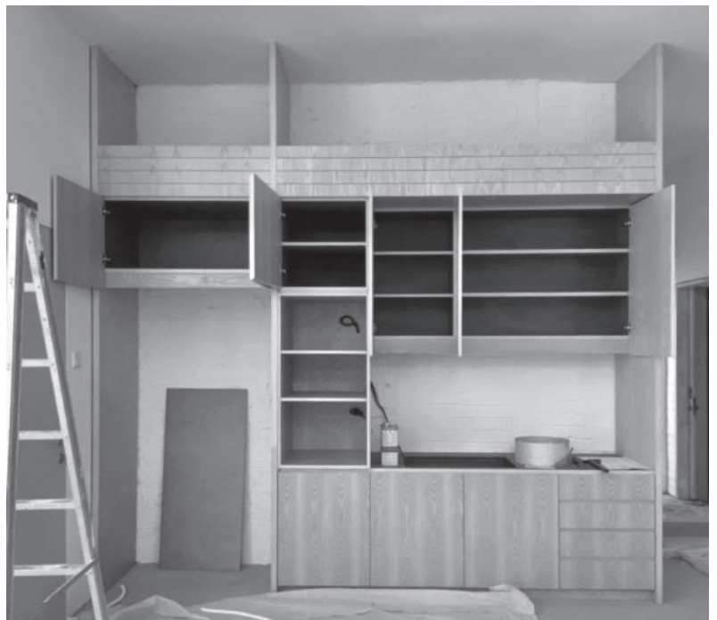
Furniture & lighting installation. (13.06.2022)
