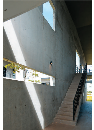
Private staircase leading towards upper floor.
