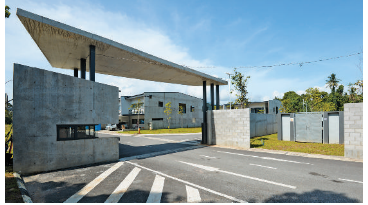
Tilted R.C flat roof at the entrance serve as an archway of the premise and provide a maintenance free shades to the guard and visitors.
