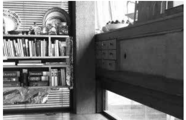
A strip of window occupies the gap between floor and hung cabinets to extend the floor plane.
