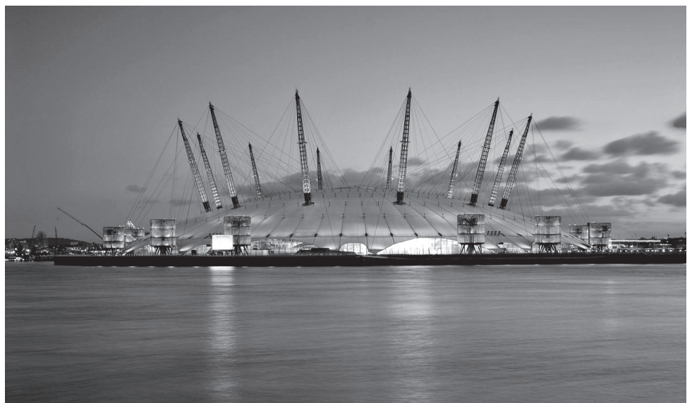
The Millennium Dome was completed in 1999 for £42 million. Its 320m diameter roof weighs less than the air contained within. (Photo: Grant Smith)
