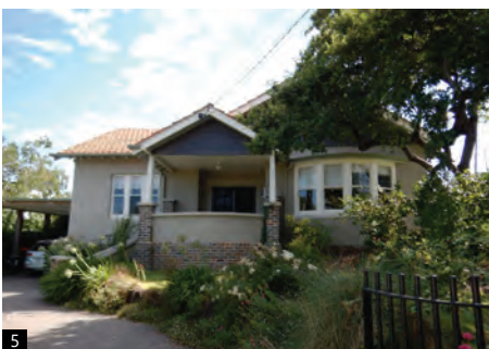
CAPTIONS: 1-4. Construction photographs. 5. View of original house from the street.
