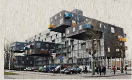
Amsterdam - WoZoCo Apartments by MVRDV.
