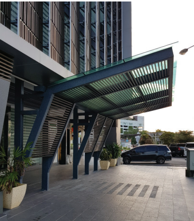
Entrance Drop-off area with overhanging steel and glass roof decorated with sun-shading louvres.
