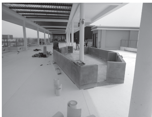
Rooftop bar in the making.
