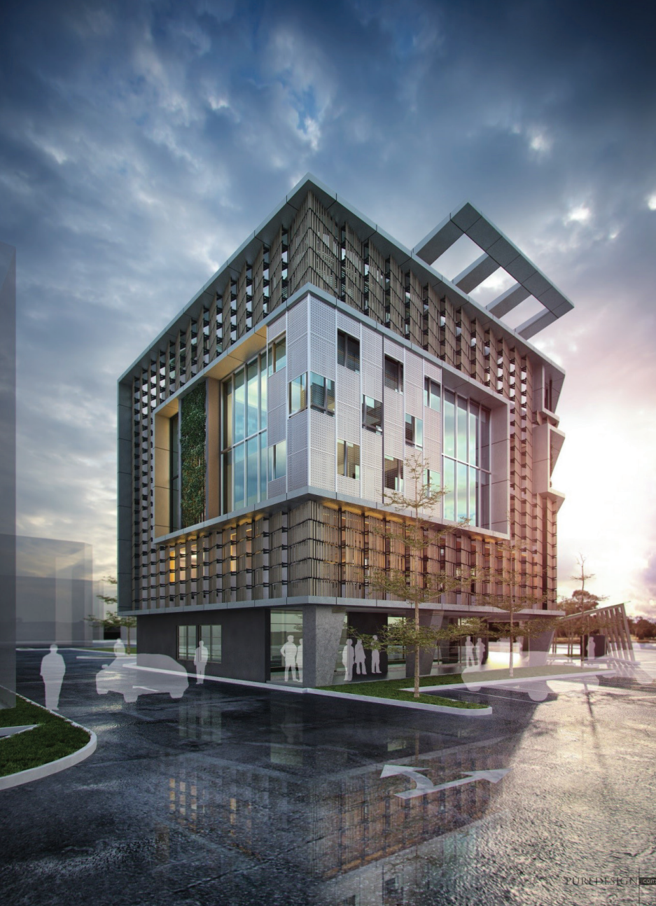
View of Building from Eastern approach. Façade panels arranged to sift off excess direct morning sunlight.
