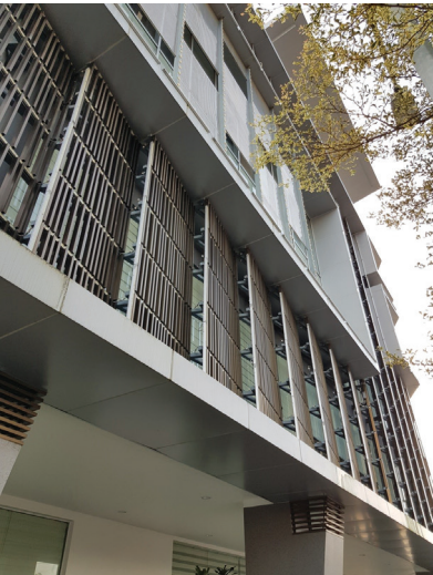
Close-up of exterior louvre panels and stainless steel mesh screen.
