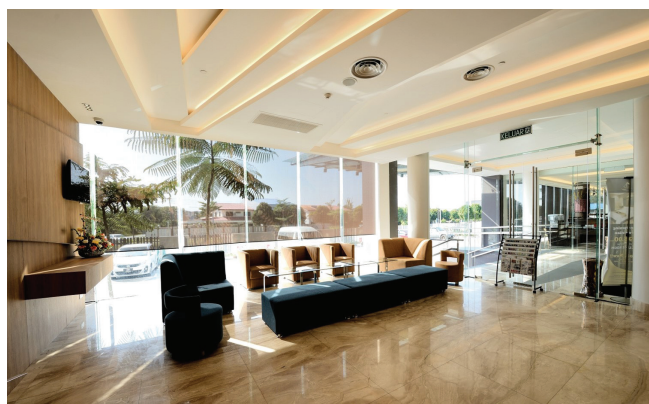
Large frameless glass panel were used at hotel lounge to bring in natural lighting with clear views.
