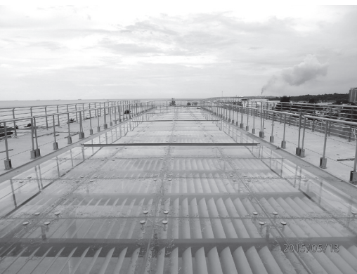
Glass canopy with louvers to screen off the direct sun light.
