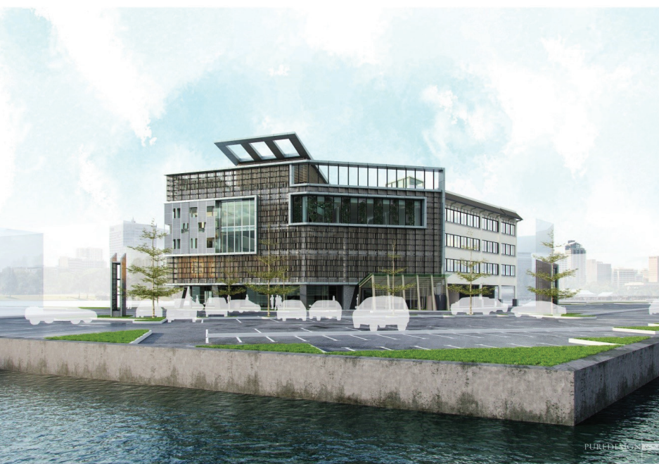
View of Building from Western approach facing the mouth of Miri river. Façade panels orientated to screen off/decrease extreme afternoon sunlight.
