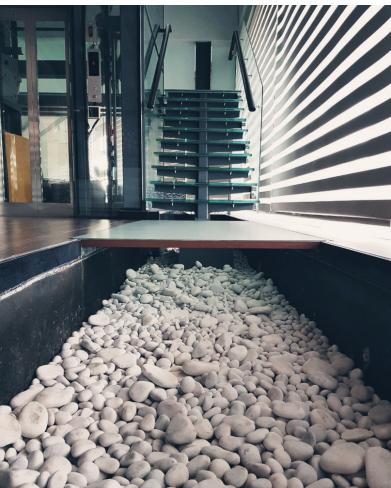
Hardscape meeting steel and glass elevator and staircase core.
