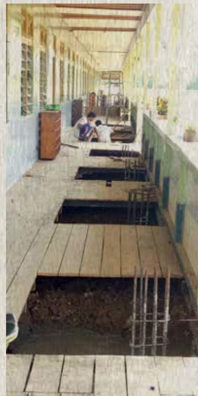
The flooring will become the permanent formwork for the new concrete floor.
