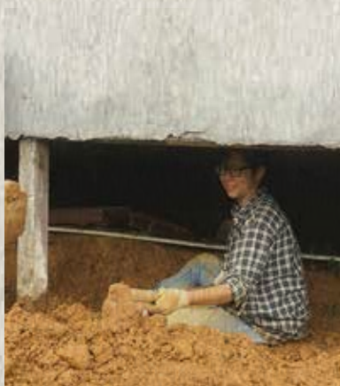
Digging the holes for new pad footings at the building's rear.
