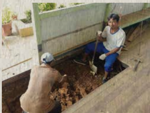
The existing timber flooring was opened up to cast footings.
