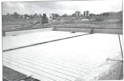
CHILDREN POOL BUCHTAL TILING IN PROGRESS
