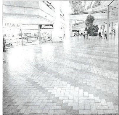
Homogeneous Floor & Granite Tiles of Subang Parade Shopping Complex, Subang Jaya
