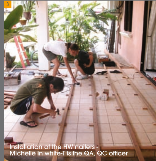
Commencement of construction - Yee Sheng and Ka Yee preparing the HW nailers
