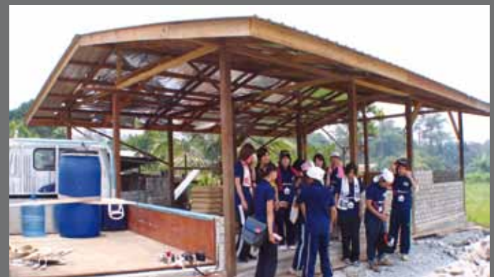
The house under construction
