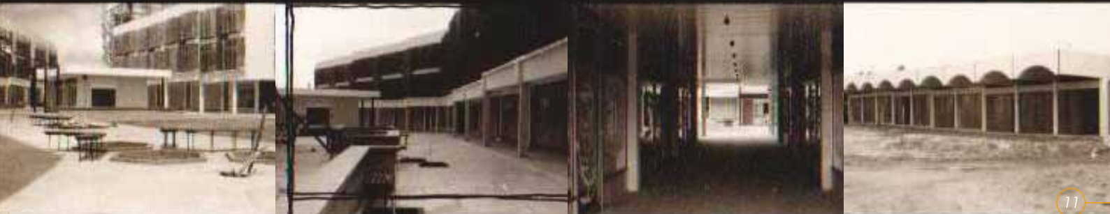
Images of Kenyalang Park Commercial Centre - Nearing completion
