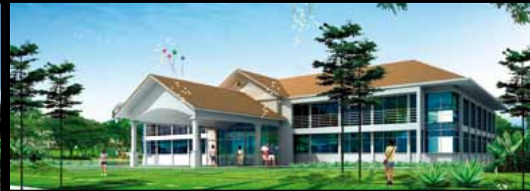
ABOVE - An artist's impression of the proposed completed SLTA Games Village LEFT - Sensitive adaptation of climate and site. These are evident in the steep gable roofs with deep overhangs, the high and low level air vents as well as the horizontally cantilevered RC ledges that span the entire building length
