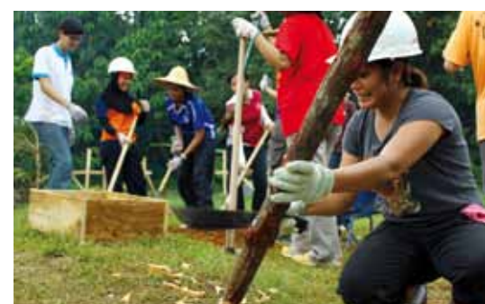
These 12 foot long piles are driven by hand.
