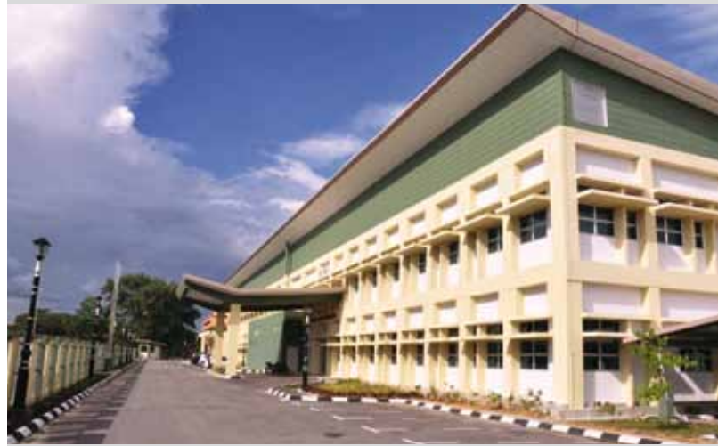
"Construction of the Klinik Kesihatan Jenis 3XP, at Bintulu, which commenced construction in March 2009 was completed in March 2012."
