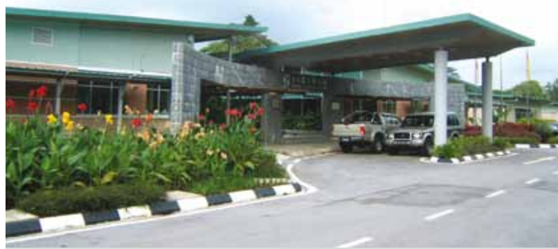
"The construction of the SBC Research Laboratories and Facilities (RM4,949,765.13) which commenced construction in January 2005 was completed in October 2005 and handed over to SBC on 13 December 2005."
