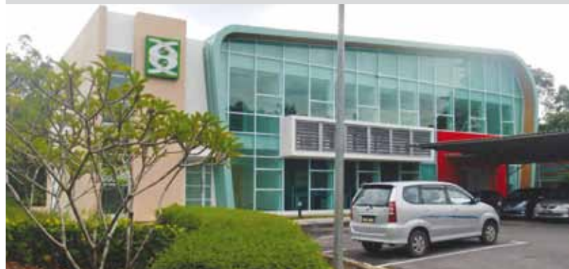
"Administrative Building of SBC Retrofitting Kuching completed in December 2009."
