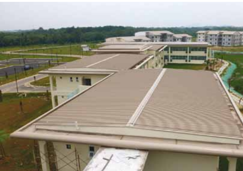
Straight and smooth bullnose facade can be achieved with detailing
