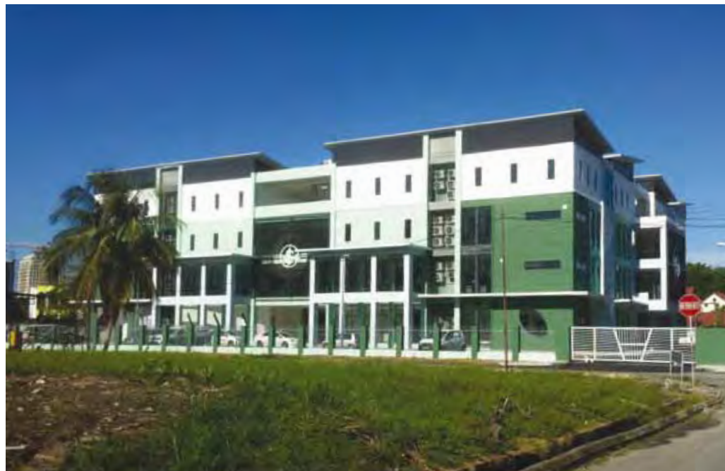
External view of the School.
