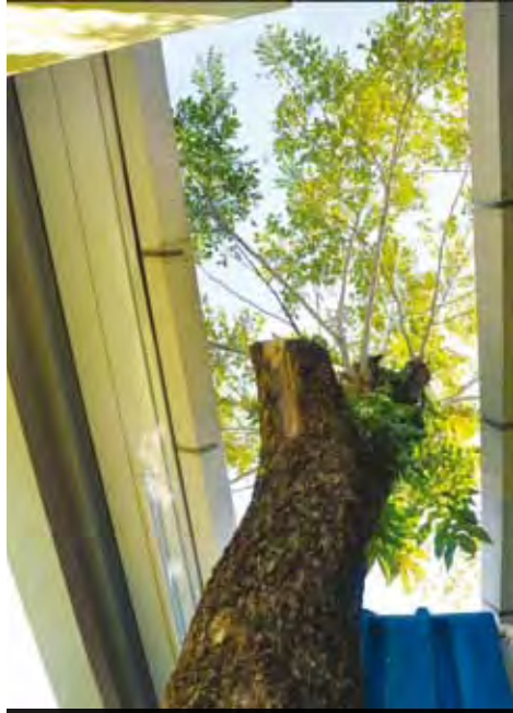
Green toilet from outside in preserving tree during construction.
