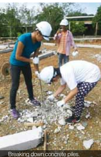
Breaking down concrete piles.
