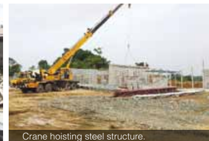
Crane hoisting steel structure.
