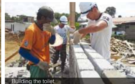
Building the toilet.
