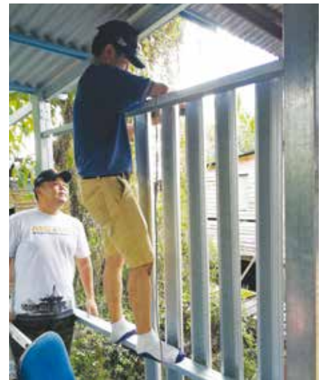
Some of the nicest details were improvised from surplus materials.
