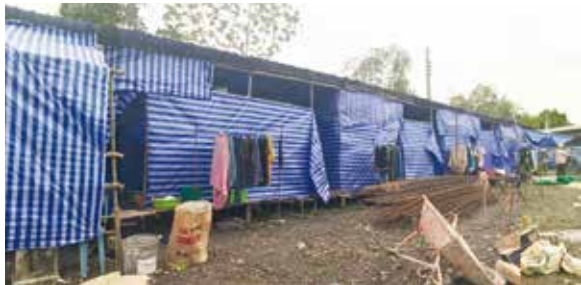
Blue canvas building - Chat equates the makeshift structures of the construction sites and temporary structures of migrants to the vernacular architecture of the past, because they suited life in the tropics and local culture. The blue plastic walls can be 'peeled back' to create a window for the inhabitants who would do most of their activities on the floor.
